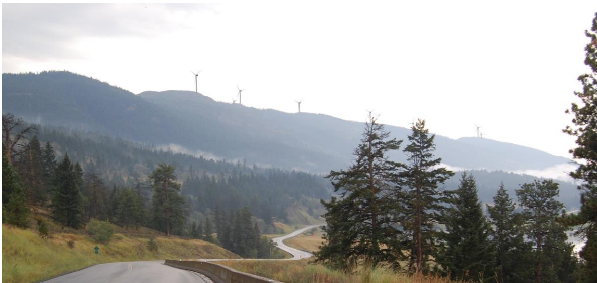
Mamette Lake Project - eight turbines* viewed from North of the project area on Highway 97C near Mamit Lake. Closest Turbine is approximately 3 km away. Looking South
